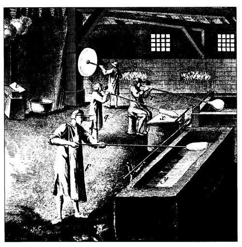
25 The manufacturing of crown glass. In front of the picture can be seen a blower lengthening the molten glass. Beyond him another blower shapes his glass on the marver. The third blower (r) shapes the glass into a globe while the fourth (s) spins the glass to open it into a table of crown glass. Note the shields worn to protect the faces of the blowers from the heat. Denis Diderot, Pictorial Encyclopedia of Trades and Industry, Plate 236.
